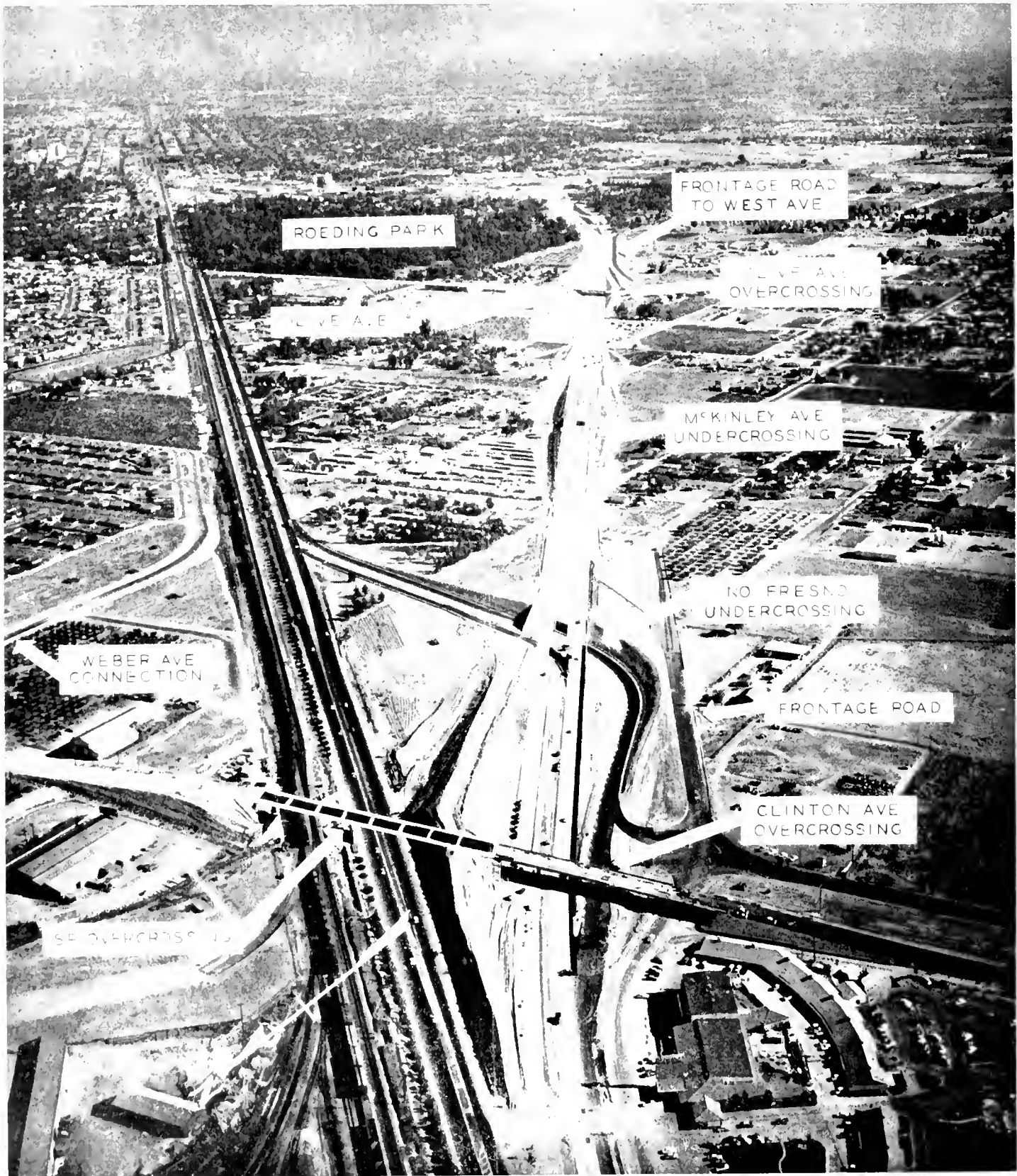
This aerial view of the Fresno Freeway shows the progress made to date on the new route which will bypass Fresno. The photograph is looking south from a point over Princeton Avenue.
